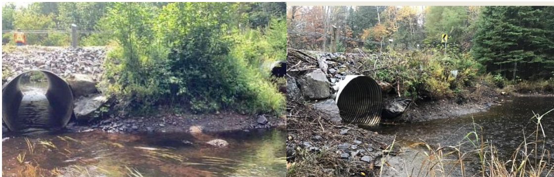
Figure 27 Eel's Lake Road Culvert (BCI=58 Fair)
