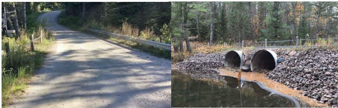
Figure 27 Eel's Lake Road Culvert (BCI=58 Fair)
