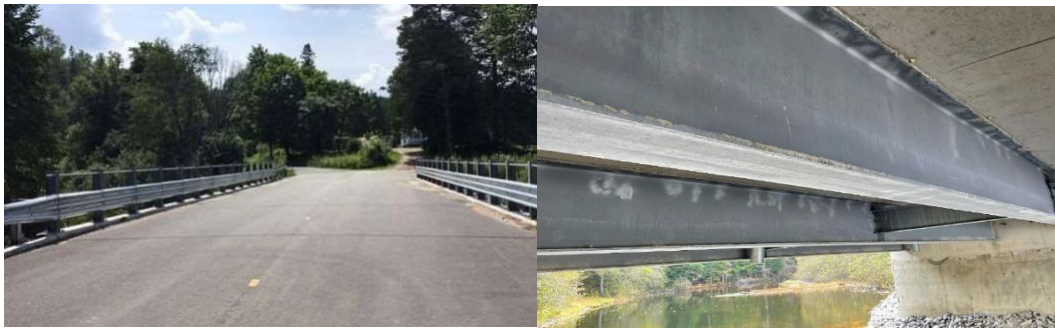
Figure 25 Tall Pines Bridge (BCI=50 Fair )
