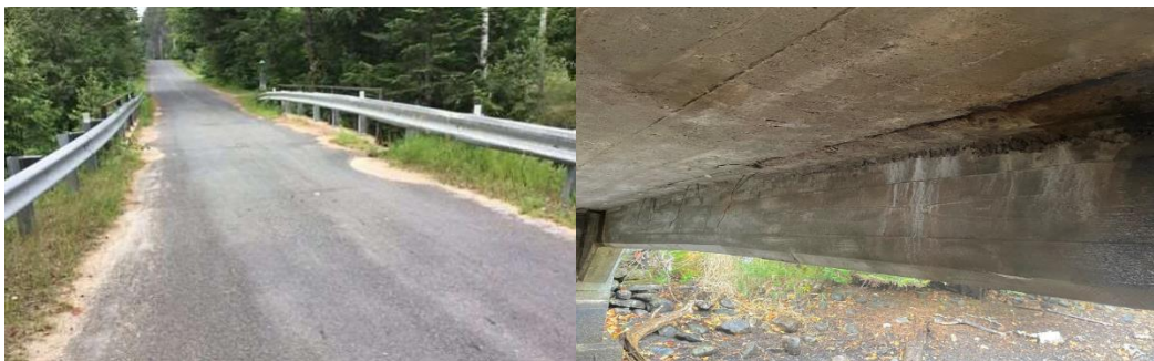
Figure 26 Universal Road Twin Culvert (BCI=80 Very Good)
